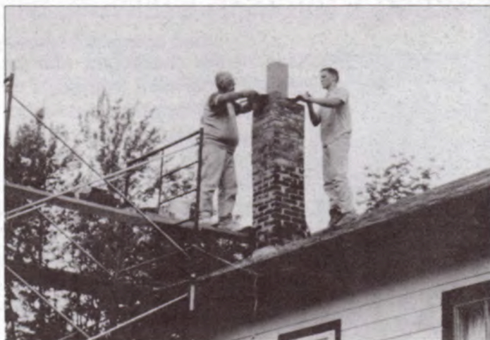
Topping out Chimney
