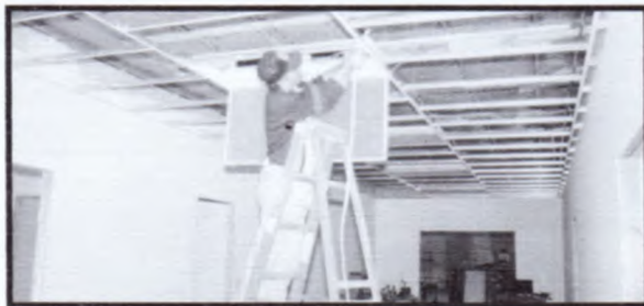
Don Delia- wiring lights
