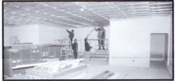
Men from Olcott Bible Church installing suspended ceiling
