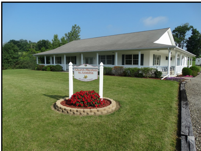
C.P.A. Headquarters Building Almond, NY
