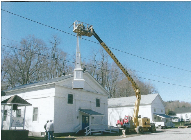
Steeple Being Installed
