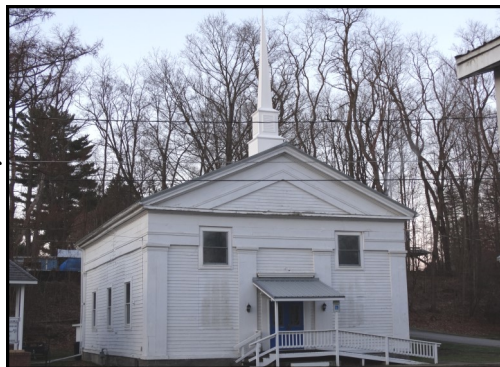
Previous Front Entrance to the Church
