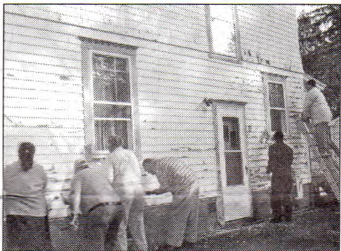
Preparing the House for Paint
