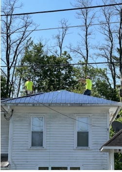
New Metal Roof
