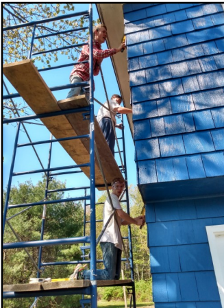
Helpers Scraping Paint
