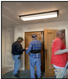
Renovating the Foyer
