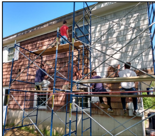
Cedar Shakes being Scraped and Primed
