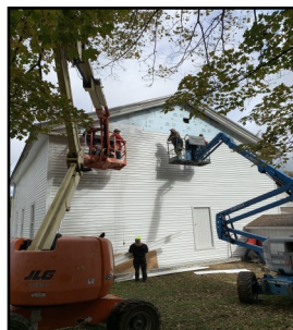
Siding on thBack of the Church
