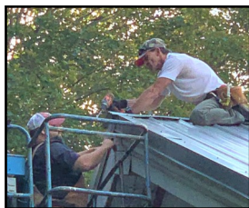
Fellowship Hall Roof Repair
