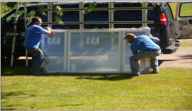
New window being installed in the parsonage!
