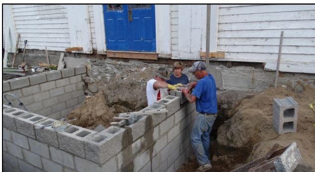
Blocks being Layed
