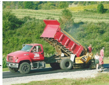
Finish Layer Being Applied
