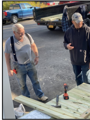
Building the Ramp
