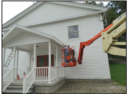
Finishing the Siding on Front
