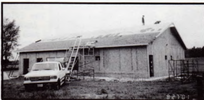
The Roof Gets Shingled
