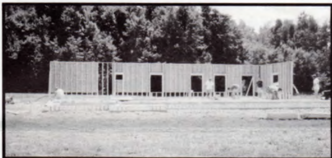
The Walls Go Up
