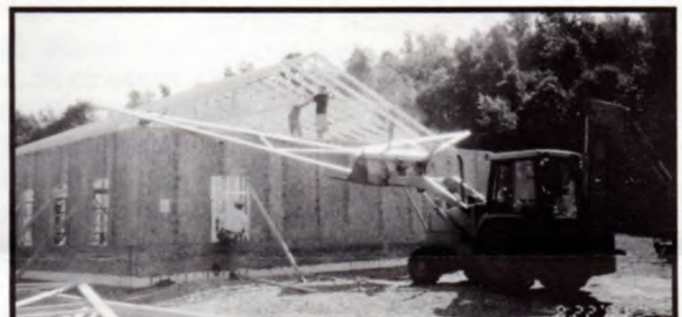
The Trusses Put In Place
