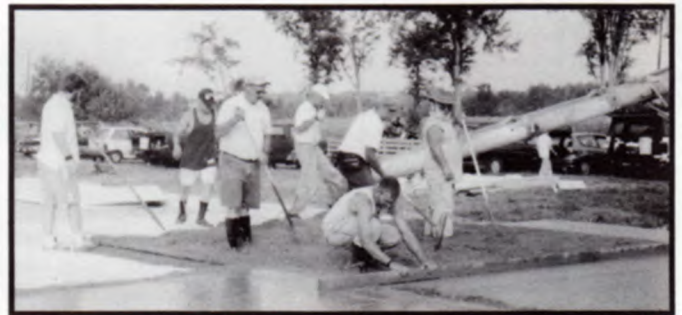
The Cement Goes Down
