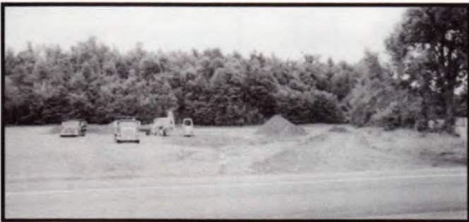
The Work Begins
